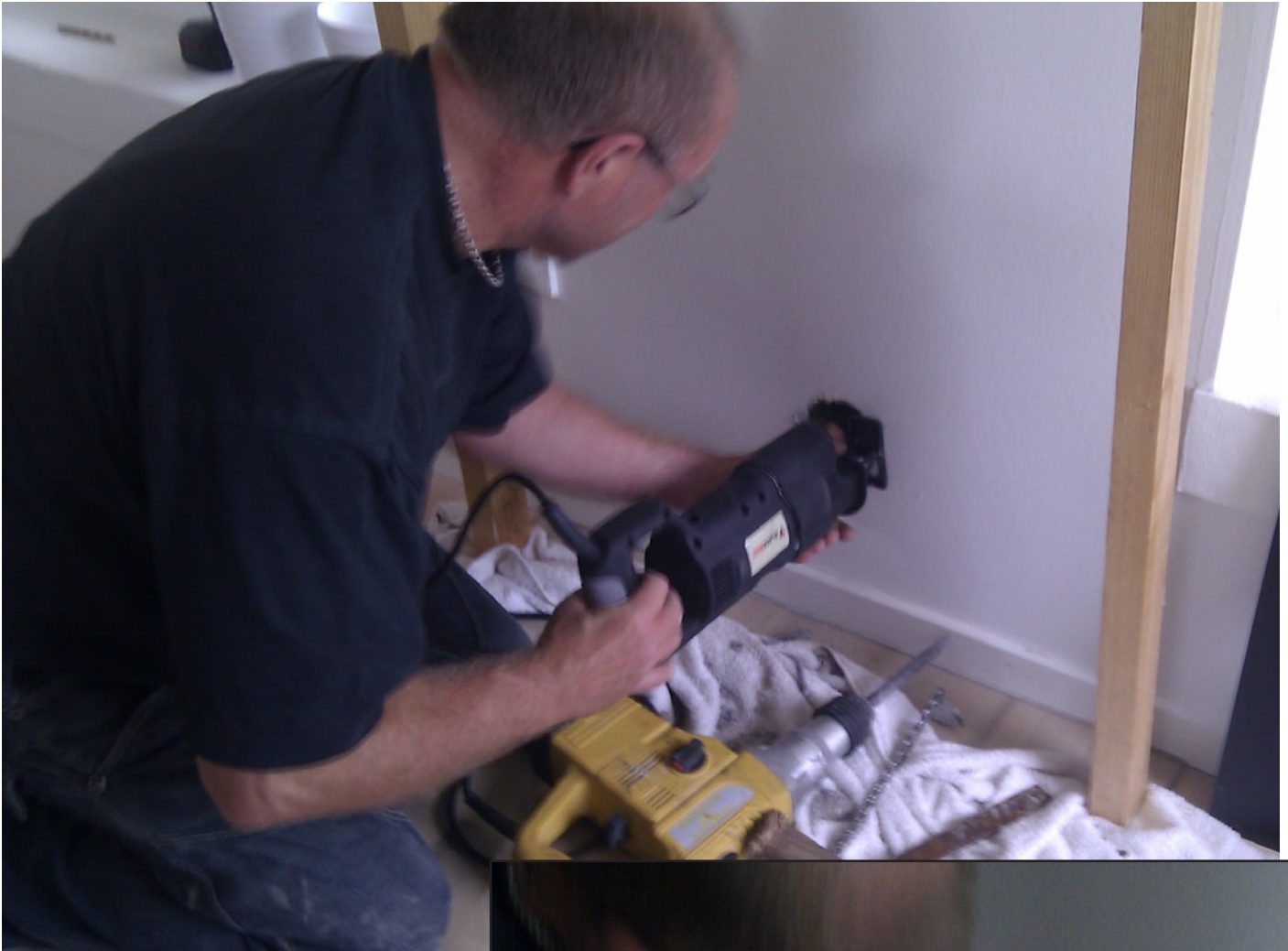
5: The reinforcement was removed with a jigsaw.
