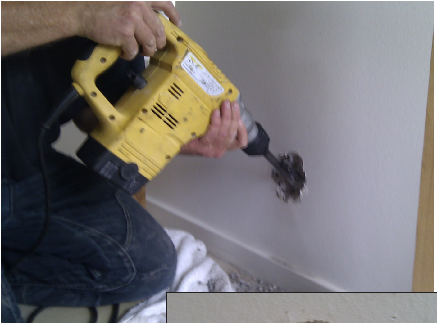
4: ... and then remove the concrete with a pneumatic drill
