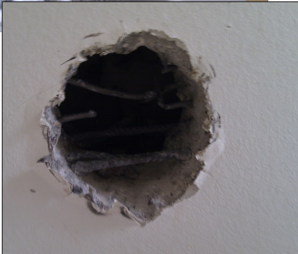
4: ... and then remove the concrete with a pneumatic drill
